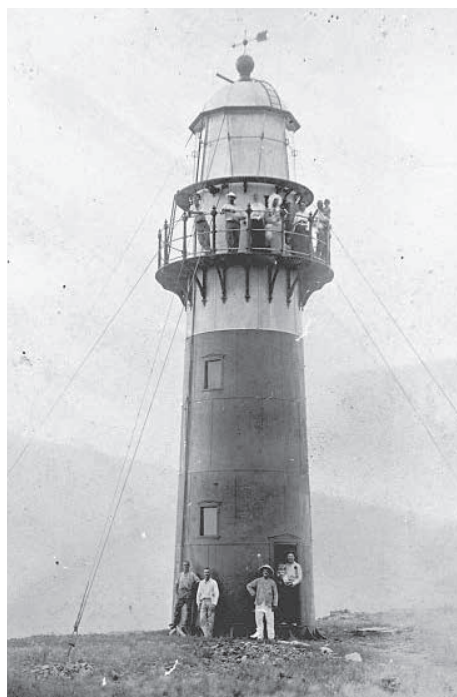
Jarman Island Lighthouse, Cossack, made of prefabricated cast iron, n.d. Courtesy Ron Richards and Heritage Council of WA (P02337)
