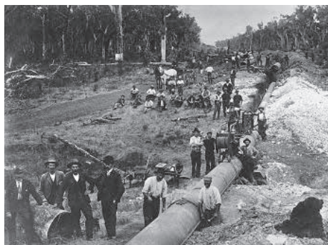
Laying Pipes across the Darling Ranges – working on the goldfields water supply pipeline, 1902. Courtesy National Trust of Australia (WA).
