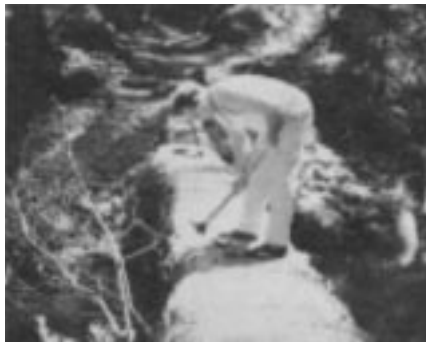
Mr. M. Coffey, preparing log for the bridge using traditional methods.
